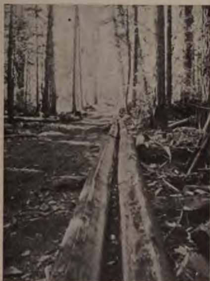
FIG. 63. — View down a Timber Slide. Idaho.
